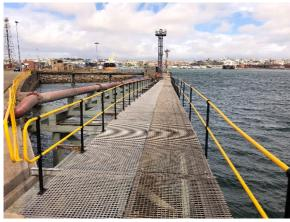
The Tanker Berth's access walkway where the corroded steel structures were repaired. The repairs entailed strengthening of the vertical columns by installation of additional vertical I-sections connected to the existing steel piles under and above water.
