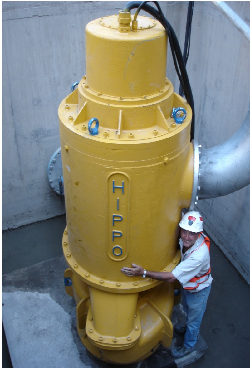
The HIPPO Med/High Voltage; High Head High Volume Flameproof Submersible Slurry Pump
