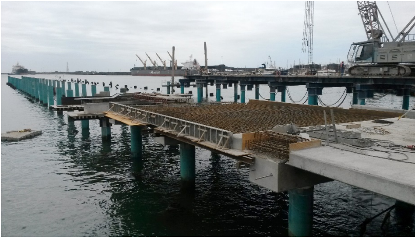
Lead-in jetties under construction.
