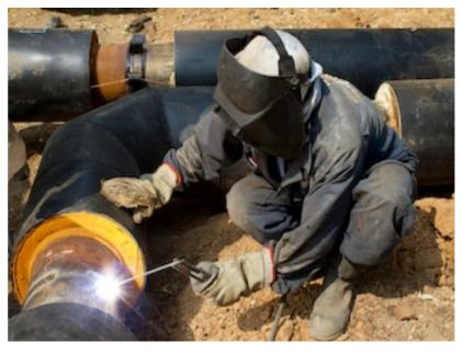
"A good weld is of paramount importance to ensure a good installation. However, owing to the fact that conditions change from site to site and the ever-present possibility of poor quality from unethical suppliers, we felt it necessary to qualify welding procedures and jobs in line with SANS 10270:2015 standards. This is in line with our mandate of ensuring a consistently high standard of fabrication and installation and ensuring peace of mind to customers," Smart clarified.
