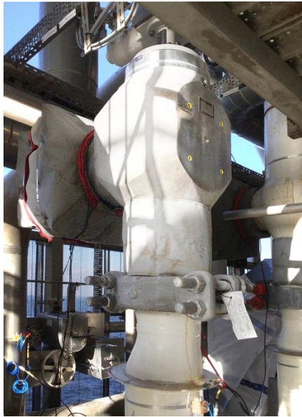
Mokveld's Angle Typhoon Valve System at Oceberg C
