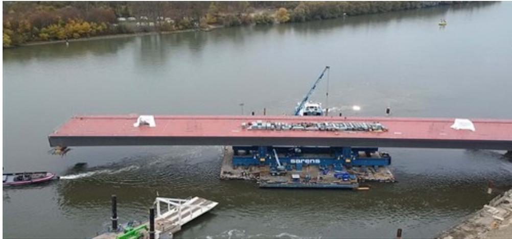
Sarens is excited to announce the debut of the CS1000 jacking system, which was used to install a 2.000T, 120-meter long segment of the new Schierstein Bridge in Germany.
