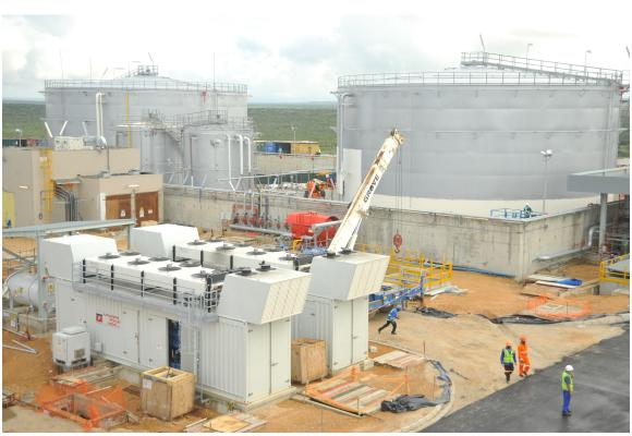
ENERGY HUB: THE Dedisa Peaking Power Plant, a liquid fuel open cycle gas turbine with a 342-megawatt (MW) generation capacity is located in the Coega Development Corporation (CDC) in Nelson Mandela Bay. Last month (June) Dedisa PPP transferred power to the national grid during a test exercise and the facility is scheduled to go online later this year. This week Coega released a tender call for a second gas-to-power plant in the IDZ.
