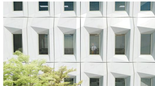
The façade is described by the project as the world's first self-supporting façade panel for construction to be made of biocomposites. Building kits for rainscreen systems, internal partition walls and suspended ceilings have also been designed and tested within the consortium funded by the European Community's Seventh Framework Programme.
