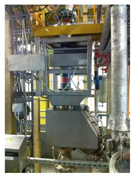
Using innovative HRF technology (High Resolution Frequency), RAPID PRO-SENSE, a system for free-fall applications, features extremely high sensitivity to all metals. (Photo: S+S)
