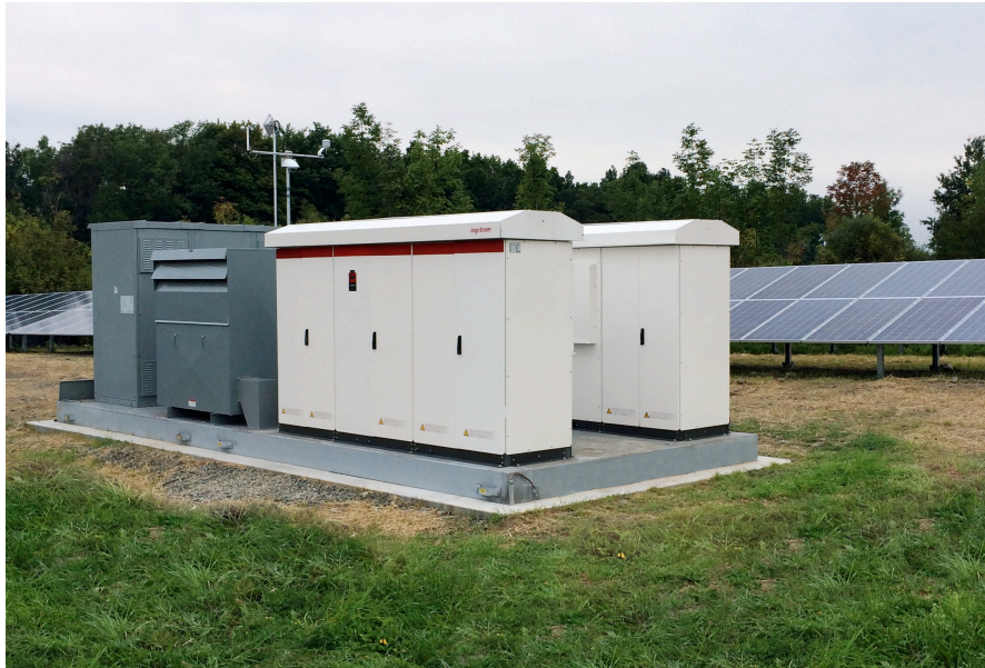
Ingeteam's power station with two outdoor PV inverters.
