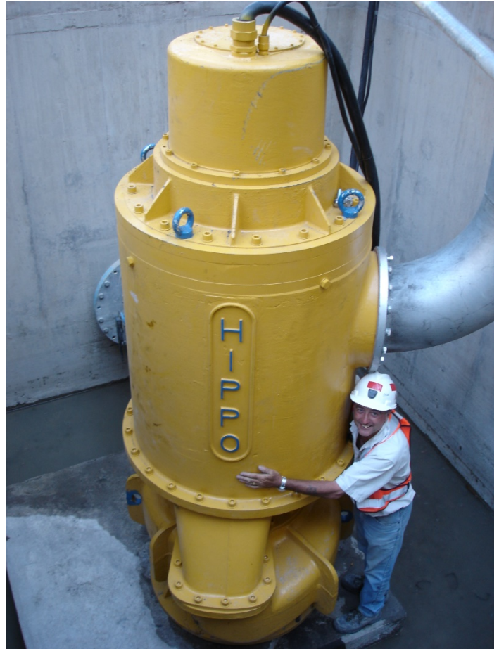
12 Ton HIPPO Submersible Slurry Pump that has been upgraded to be able to have the mechanical seals replaced on-site by the user .
